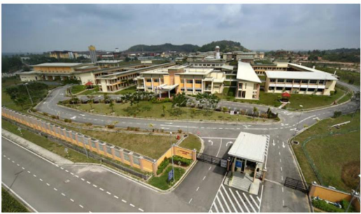
Proposed construction of a 100 ft road leading into MRSM Bandar Seri Alam, Johor Bahru. Earthworks computation, design of external sewer line and external water reticulation leading to the reservoir.
