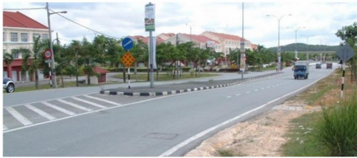
JKR Road J4 (Package B11) Jalan Lima Kedai/Gelang Patah road upgrading.
